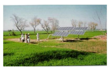
Figure 12.6 Photovoltaic Water Pumping
