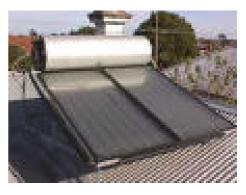
Figure 12.1 Solar Flat plate collector
